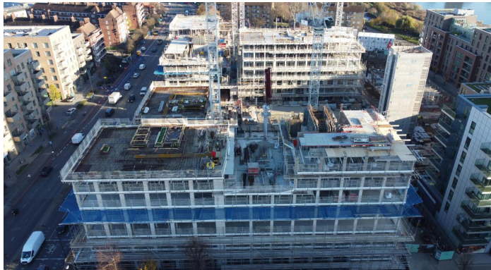
Concrete frame reaching 6 th floor level
