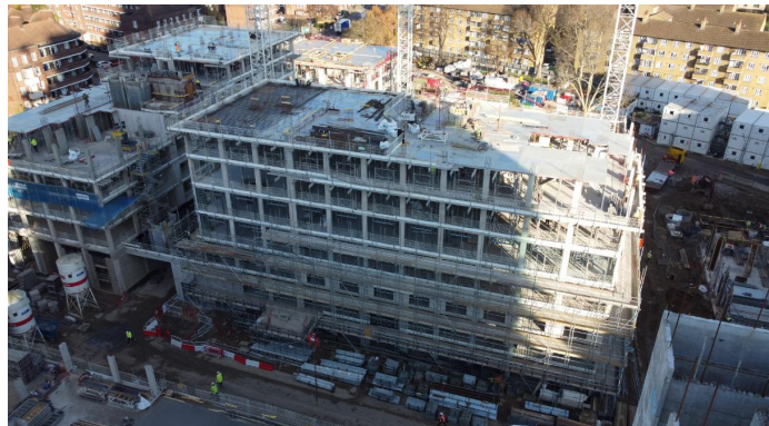
Concrete frame reaching 6 th floor level
