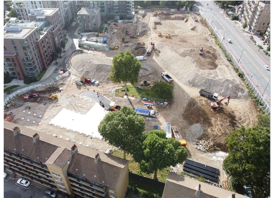
Hardstanding for the site compound is being laid
