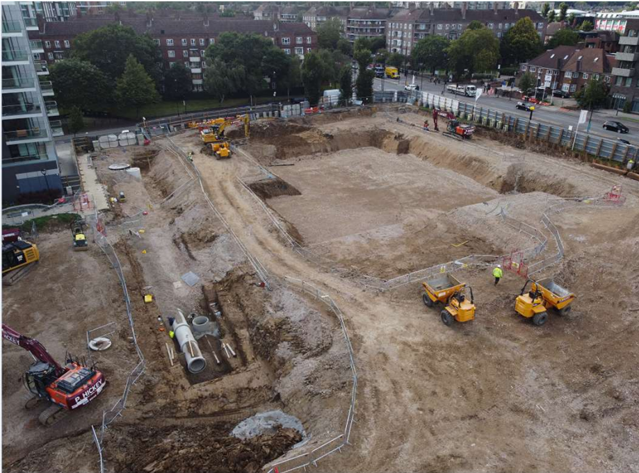
Drainage pipes are being laid
