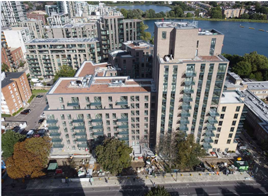
Balcony installation to Core B1 complete
