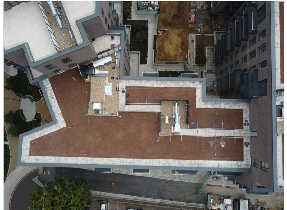
Core B3 roof works complete
