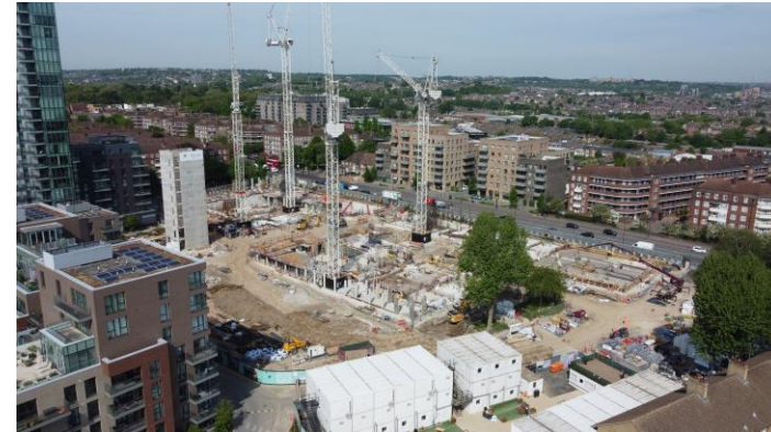
Fourth Tower Crane now in place on Phase 3
