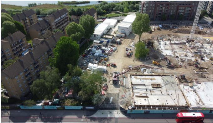
New site access off Seven Sisters Road completed
