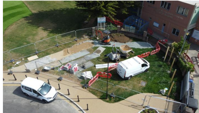
Hackney Council works providing temporary footpath to Liliput Centre
