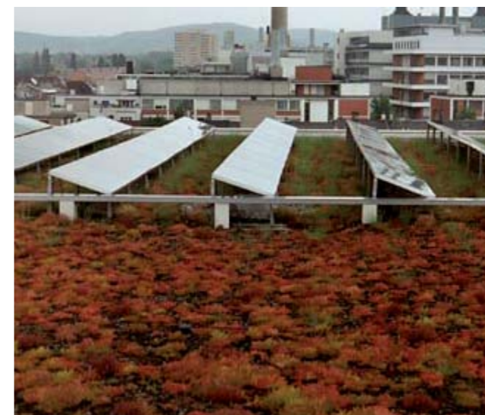
Certain roofs will combine solar panels with a brown roof habitat for Black Redstarts
