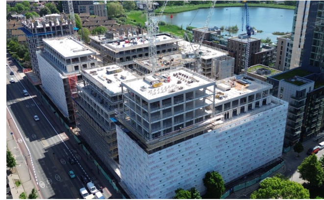
Concrete frame advancing
