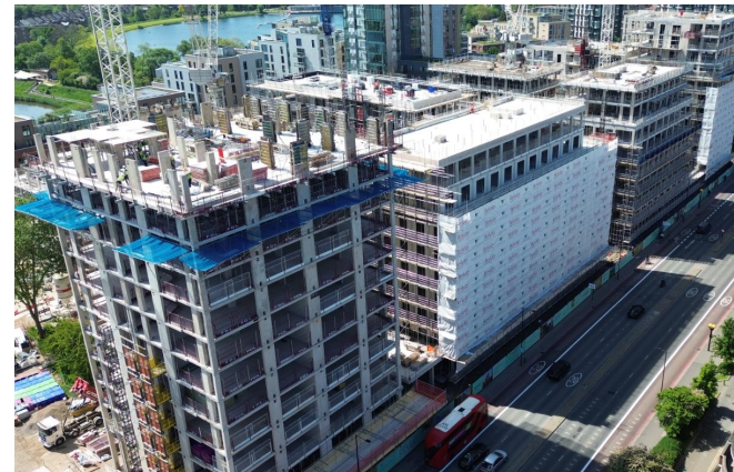
Concrete frame ongoing
