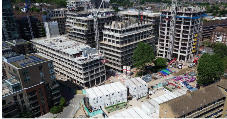
Concrete superstructure developing
