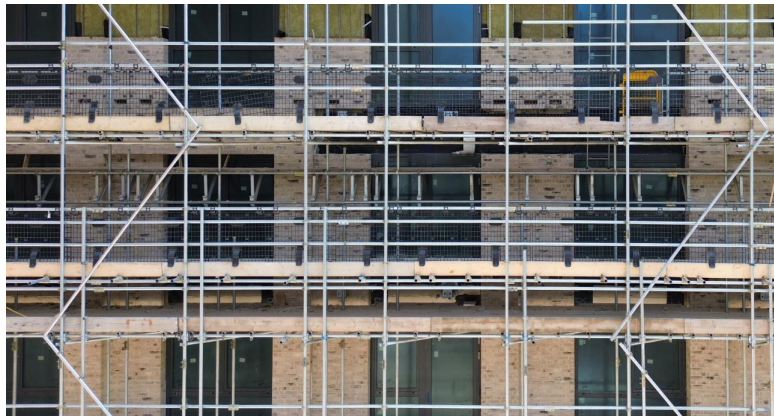
Brick work started and windows installed.
