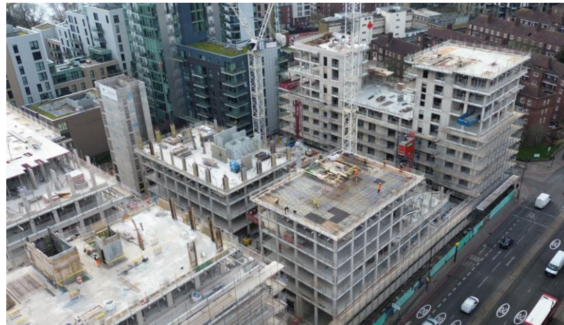
Concrete frame reaching 9 th floor level on the A Blocks
