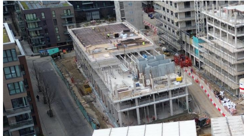
Concrete frame advancing on B4 & B5
