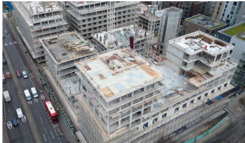
Concrete frame reaching 9 th floor level on the A Blocks
