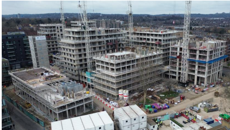
Concrete superstructure developing
