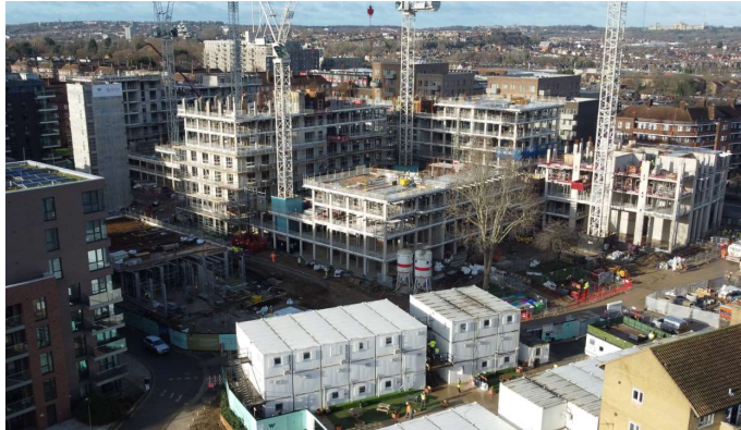
Concrete superstructure developing
