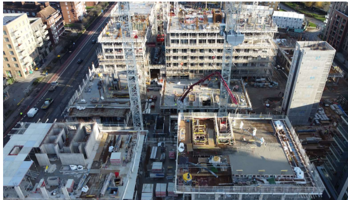
Concrete frame reaching 7 th floor level on the A Blocks
