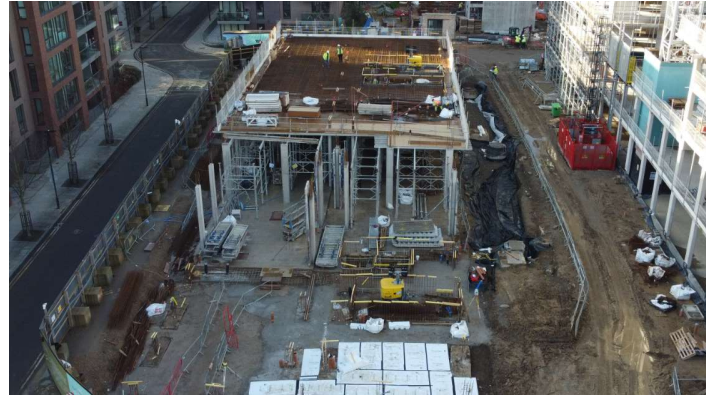
Concrete frame advancing on B4 & B5
