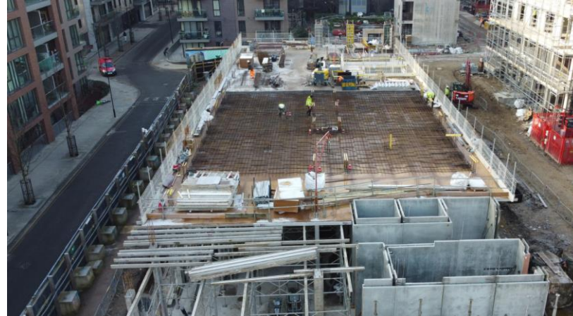
Concrete frame advancing on B4 & B5
