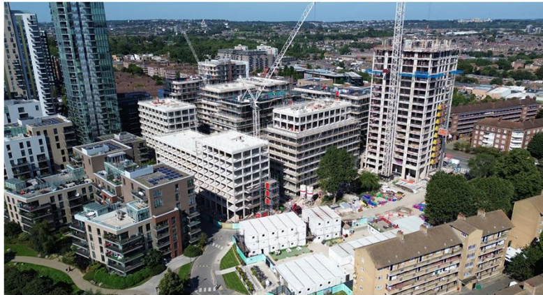
Concrete superstructure developing
