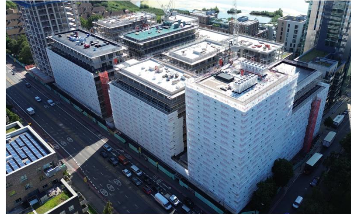
Concrete frame advancing
