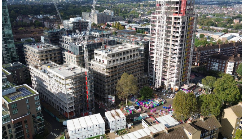
Concrete superstructure complete
