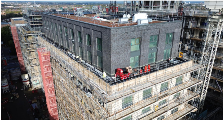
Scaffold on B6 starting to be removed.
