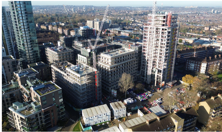
North West View
