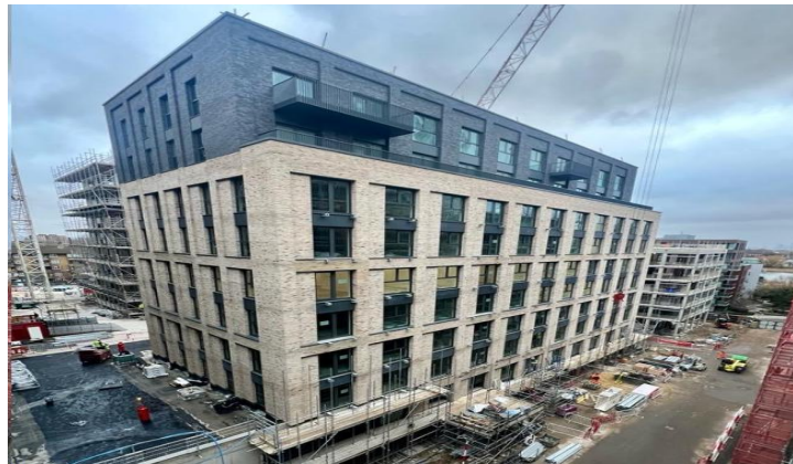
Scaffold on B6 down to Ground Floor.
