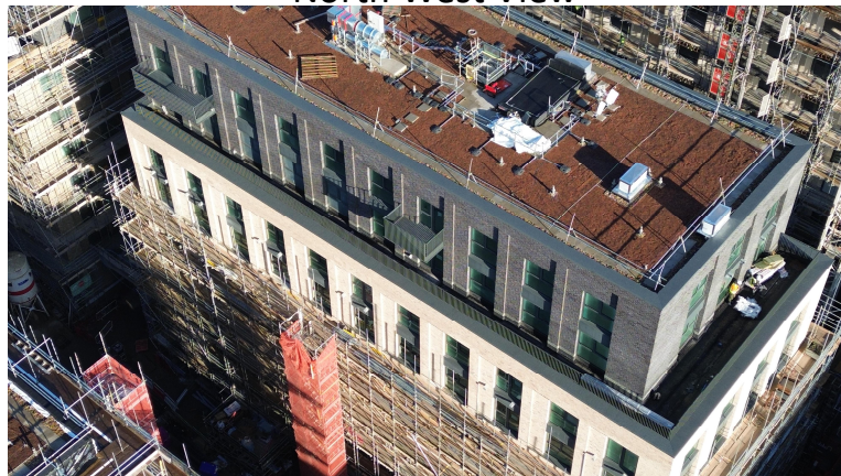
Scaffold on B6 down to 4 th Floor.
