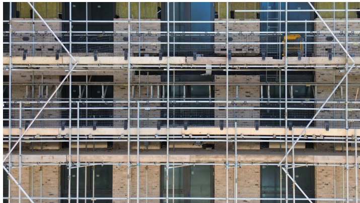
Brick work started and windows installed.
