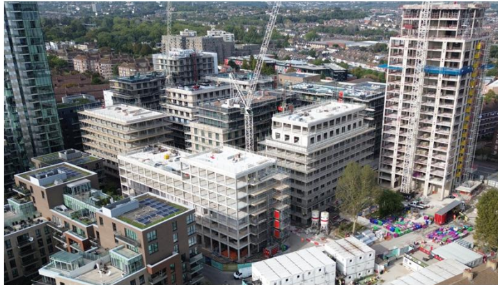
Concrete superstructure concluding
